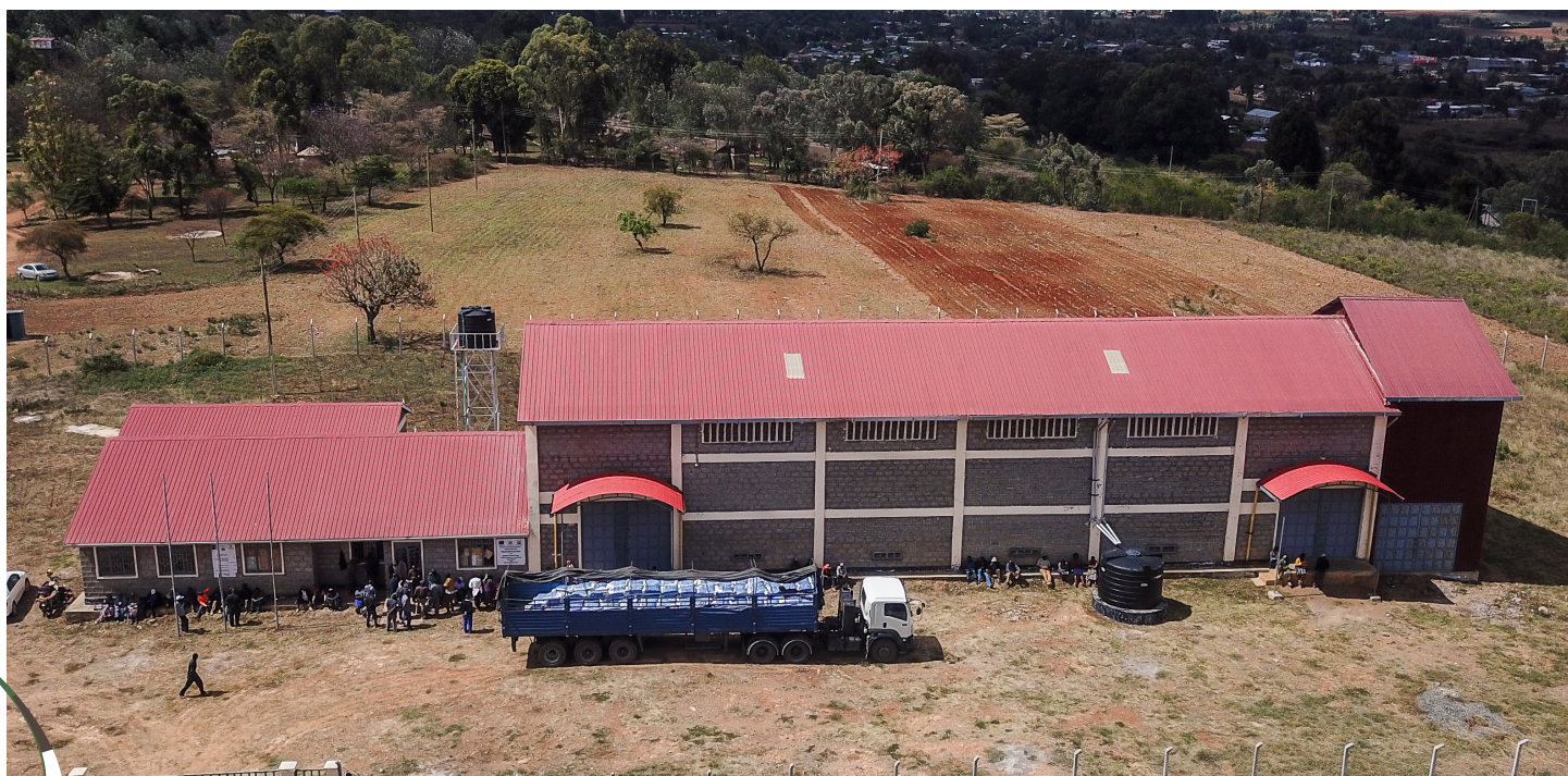
Kinamba Warehouse in Githiga ward, Laikipia West Sub-county
