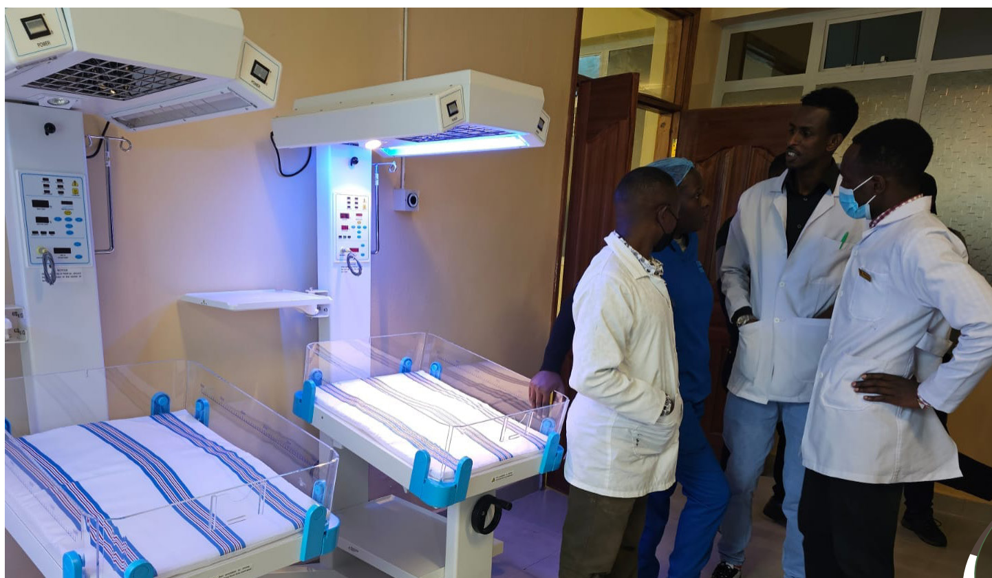
Antenatal and postnatal care; Infant warmers installation at NCRH
