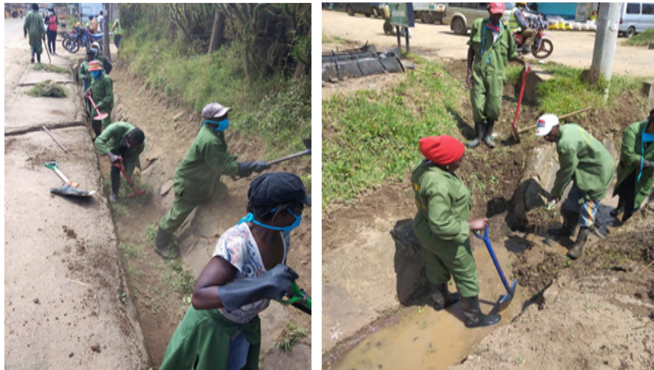
Plate 1: Unclogging and maintenance of drainages in Nanyuki town
