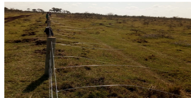
Mathira Solar Powered Human-Wildlife Fence: A total of 6.2 km of Human-Wildlife fences have been successfully installed.
