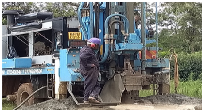
Appendix 11: Drilling of Bustani borehole
