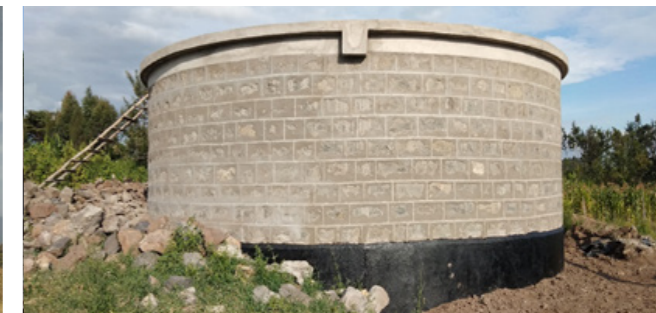
Appendix 19: Construction of a 135M3 Concrete Tank at Mikubune
