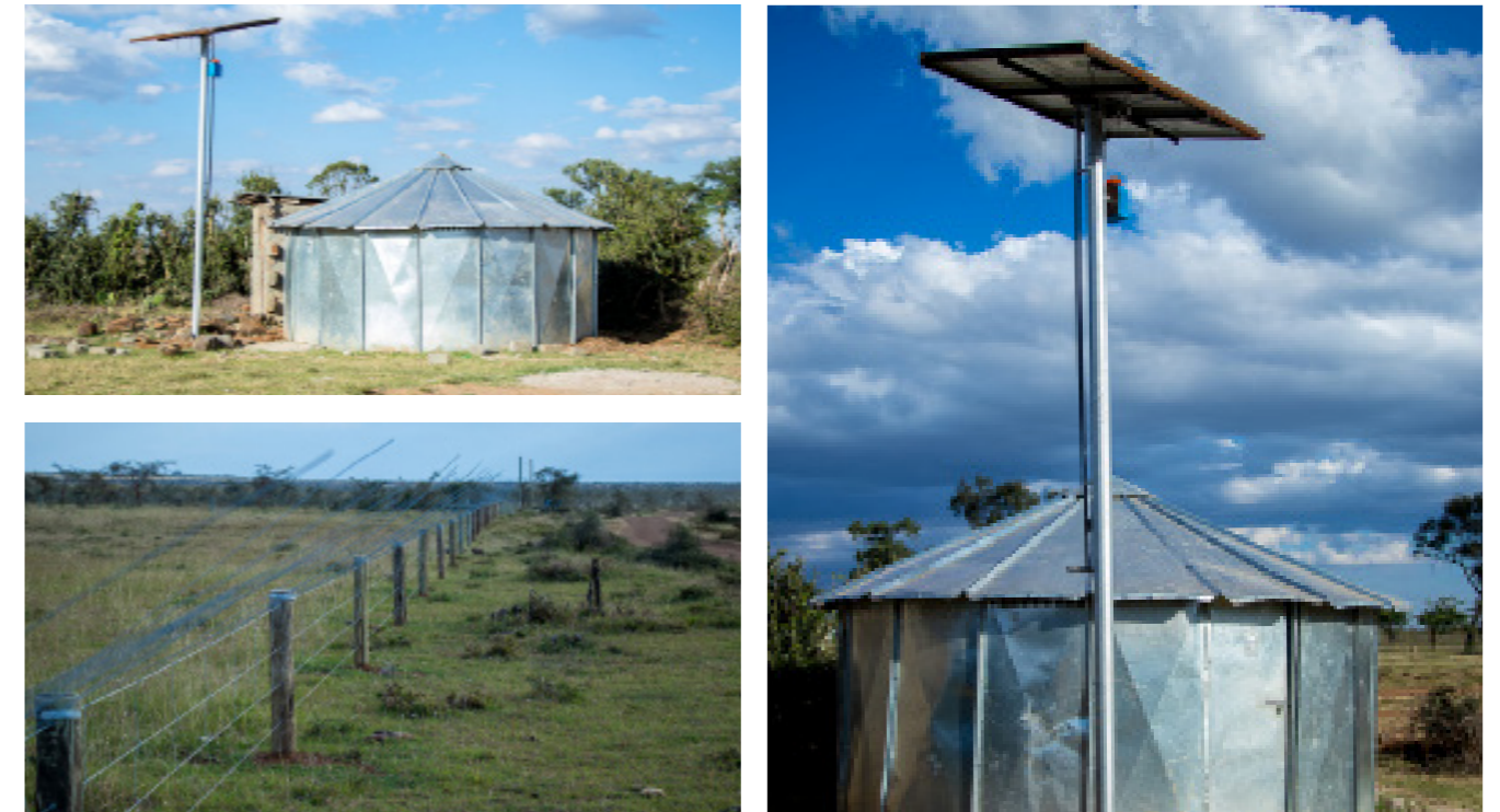
Appendix 25: Murungai borehole in Umande ward
