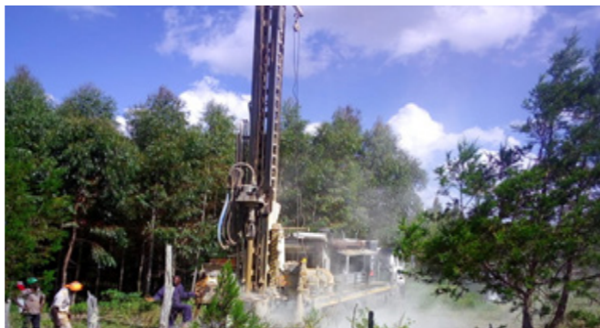
Appendix 14: Drilling of Gatitu Borehole
