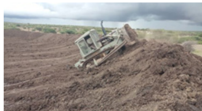
Appendix 5: Loshaki Dam rehabilitation works
