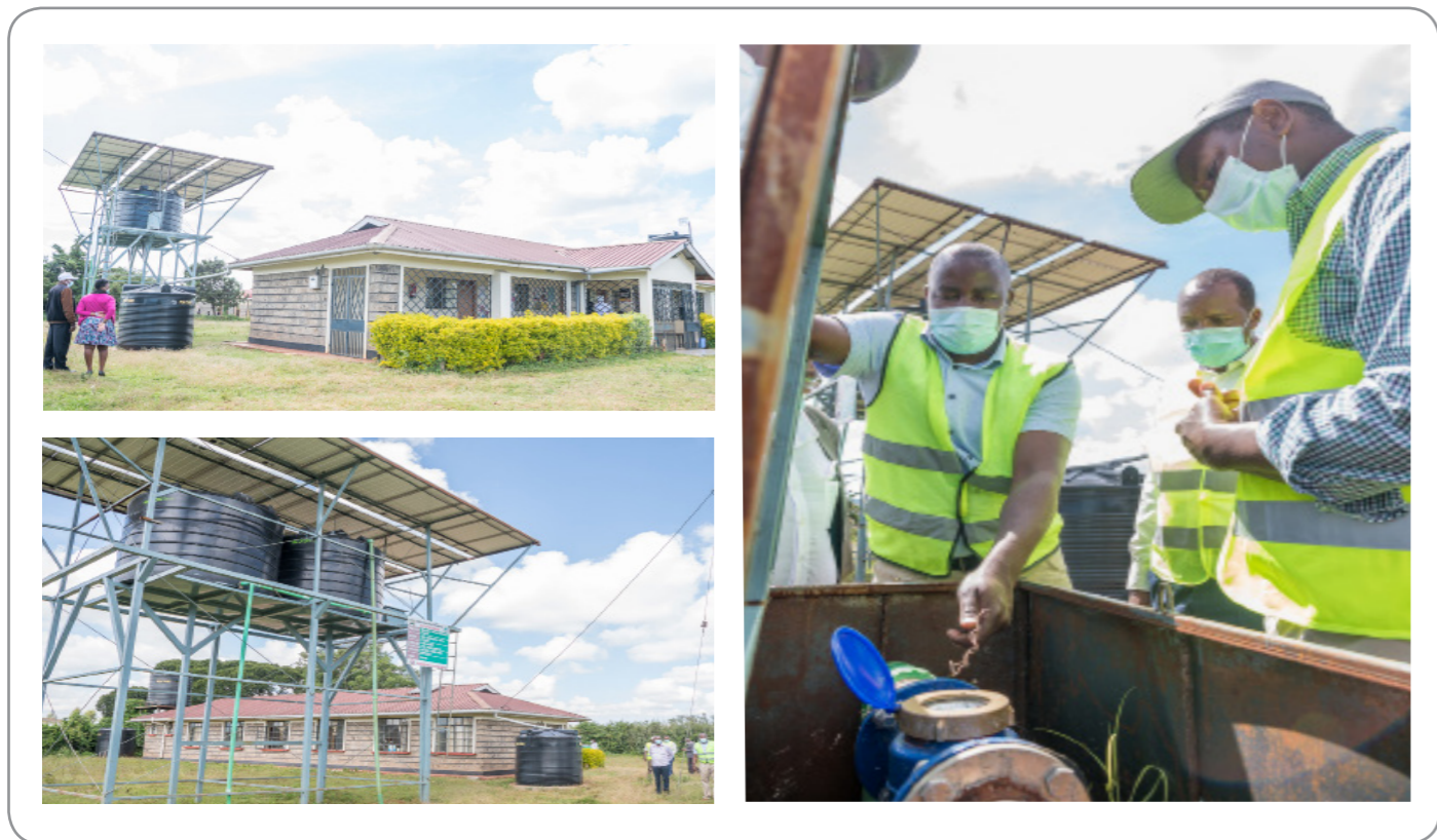
Gallery 2: Inspection of Mugumo dispensary borehole
