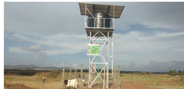
Appendix 18: Solar Equipping at Tetu borehole
