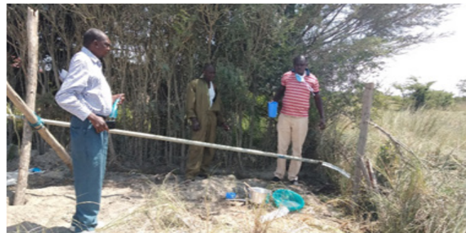
Test pumping at Yard Primary School borehole
