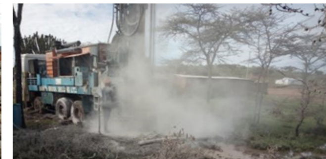
Appendix 10: Drilling of Oldigiri primary school b/h -Dry borehole
