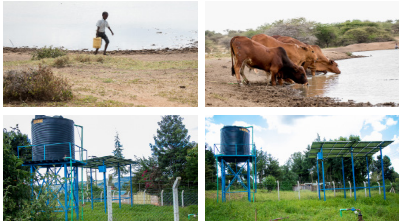
Appendix 24: Drilling and Equipping of Muthengera borehole in Igwamiti ward
