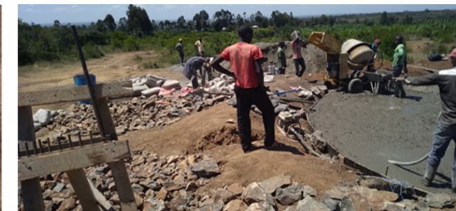
Appendix 8: Concreting of floor slab for nganoini masonry 135m3 tank
