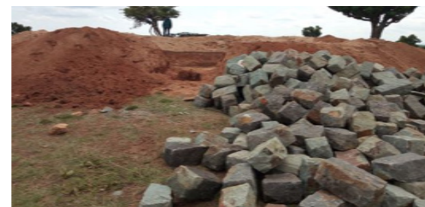
Appendix 1: Foundation excavation for the 225M3 masonry tank and materials for Osirwa W/P
