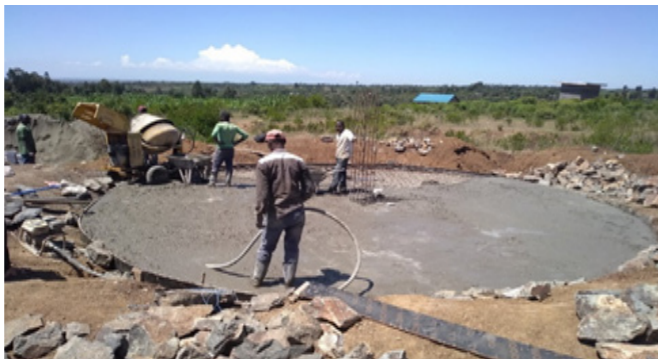
Appendix 12: Concreting of floor Slab for Nganoini Masonry 135M3 Tank
