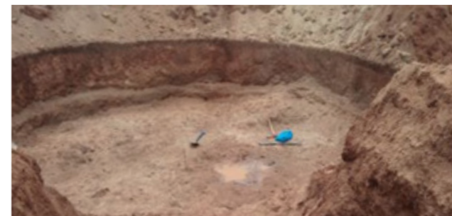
Appendix 7: Foundation excavation for the 225M3 masonry tank
