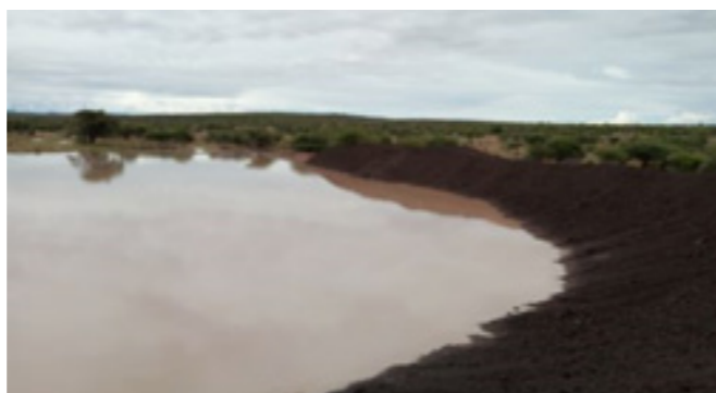
Appendix 6: Loshaki Dam after rehabilitation
