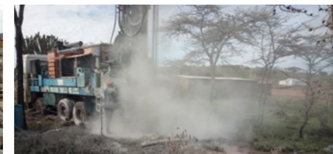
Appendix 2: Drilling of Oldigiri primary school b/h –Dry borehole
