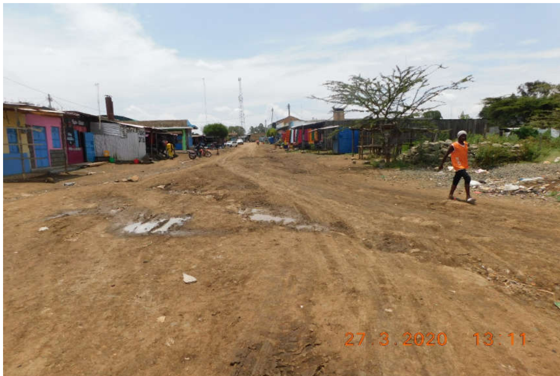
Gulleys on the road due to impended drainage
