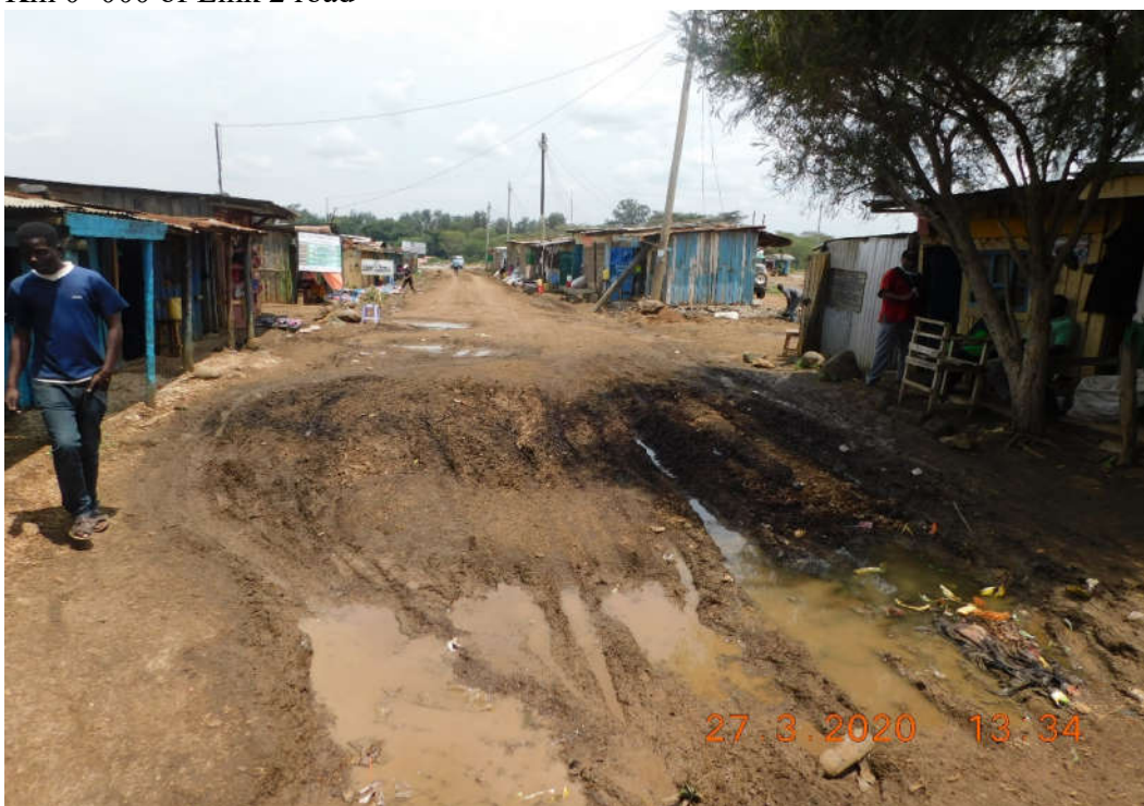
A poorly drained section of the link 2 road.
