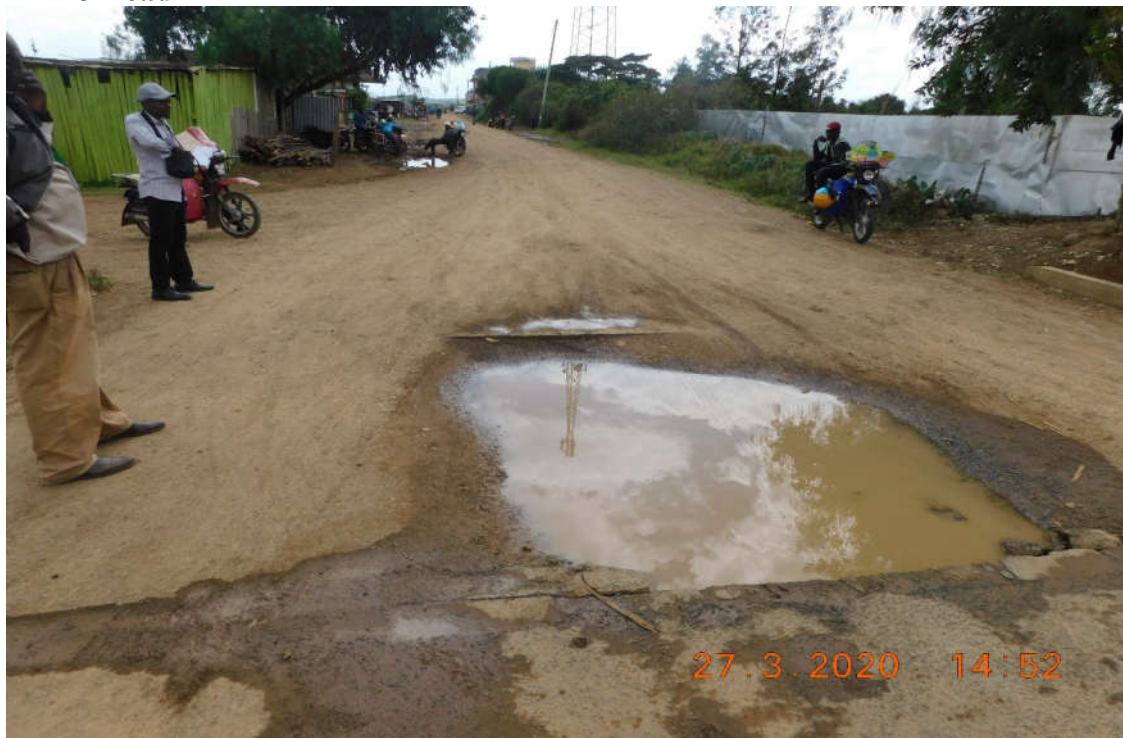
Water ponding at Km 0+000 of link 3 road
