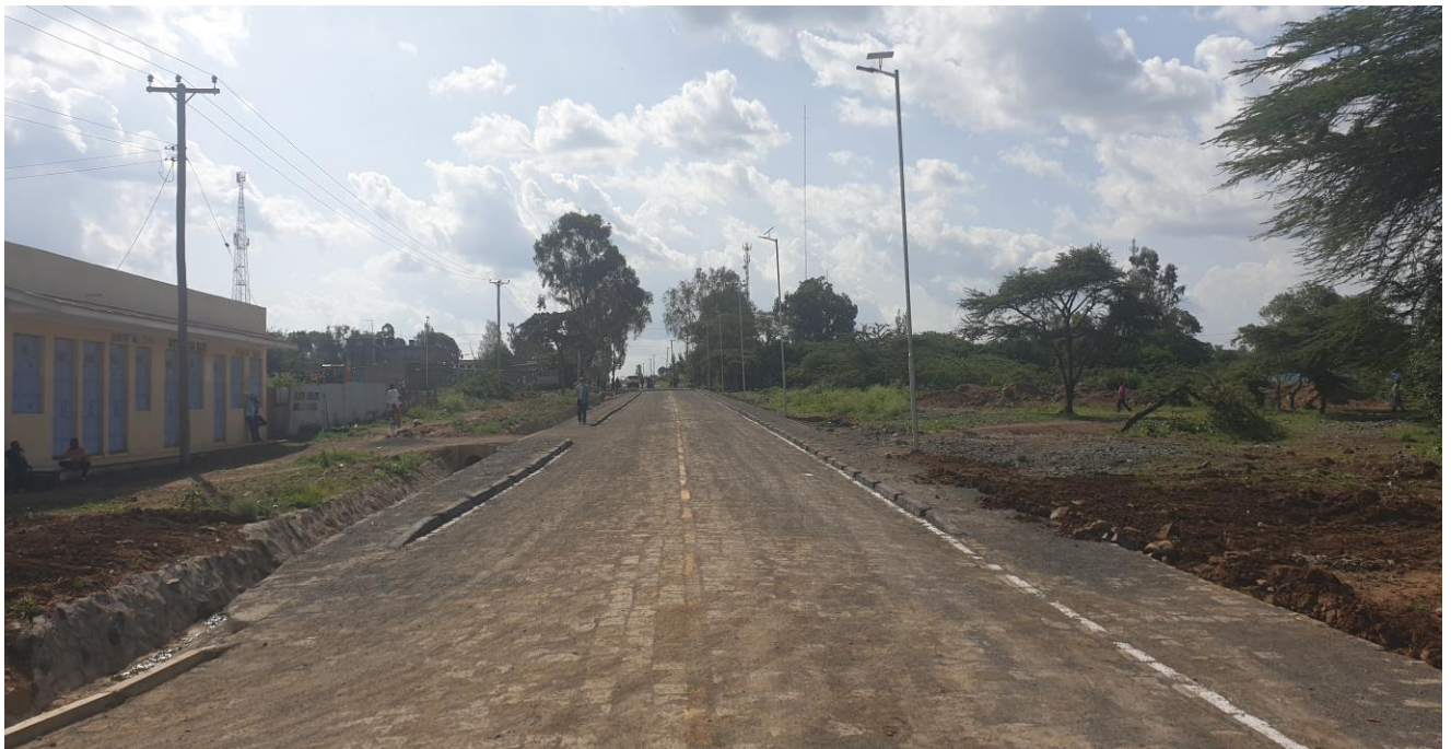
Figure 2: Completed Solomon Kiguru Road.
