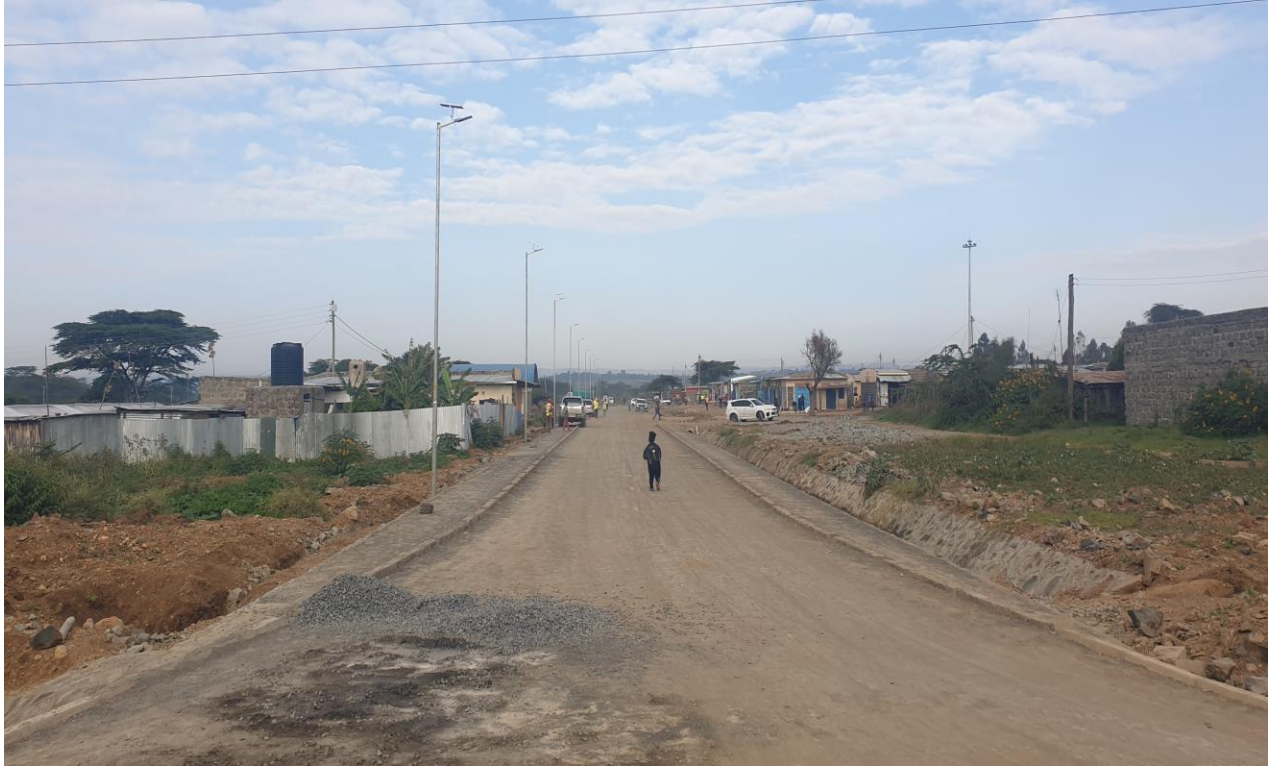
Figure 5: Completed street lighting along Kihika Kimani Road
