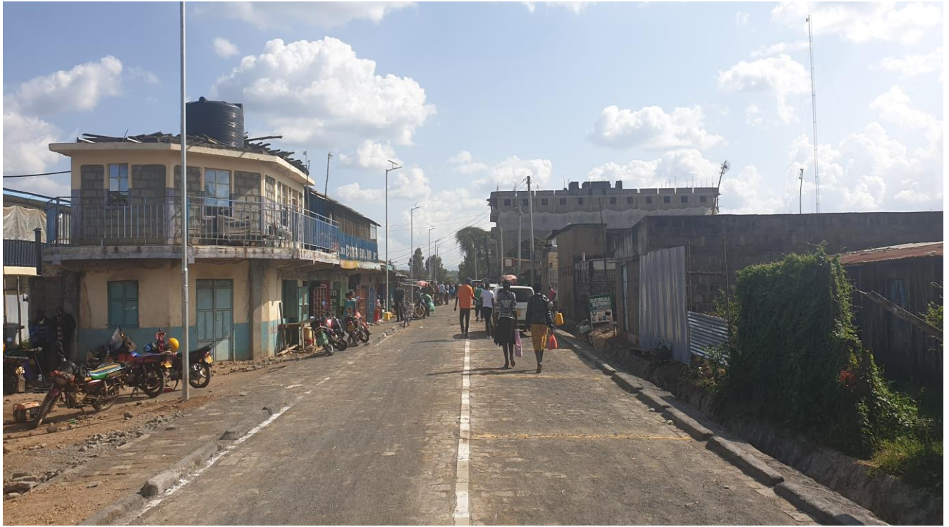
Figure 4: Completed GG Kariuki Street
