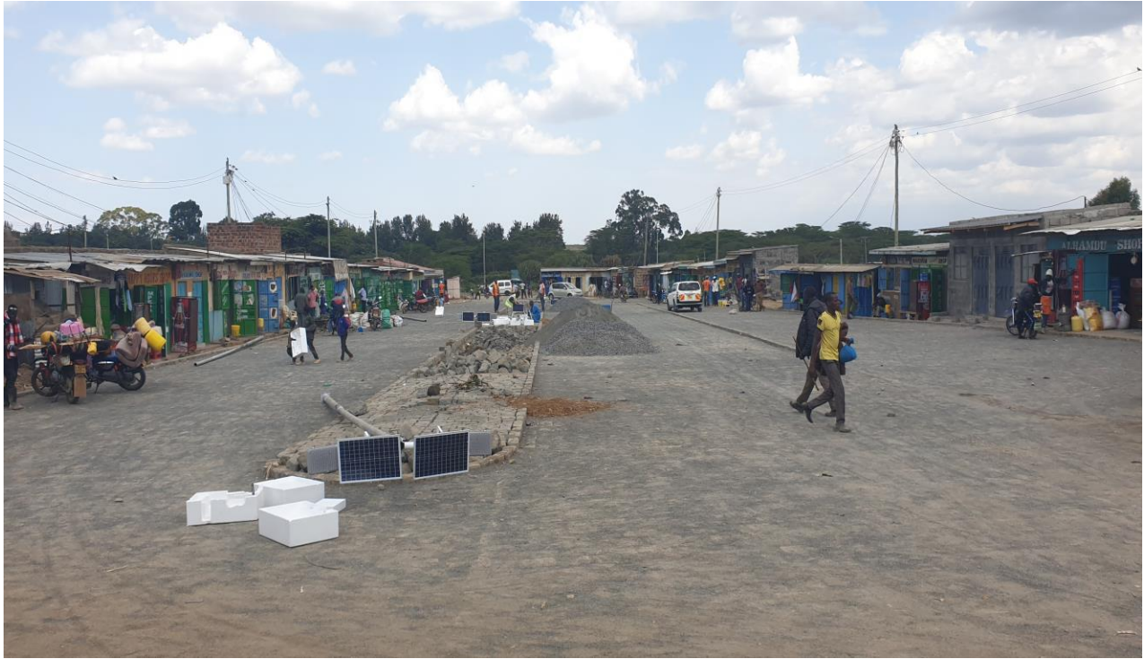
Figure 6: Installation of solar powered street lighting at the bus park ongoing.
