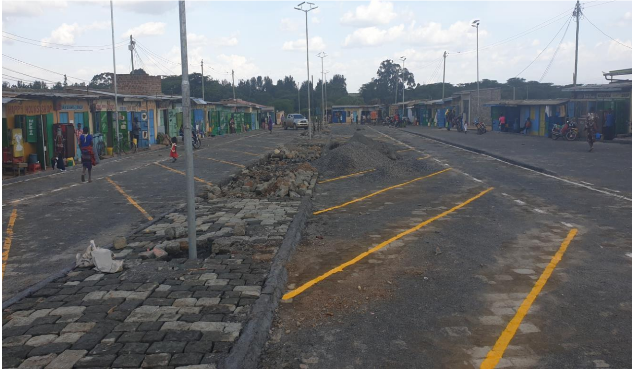
Figure 7: Nearly complete bus park.
