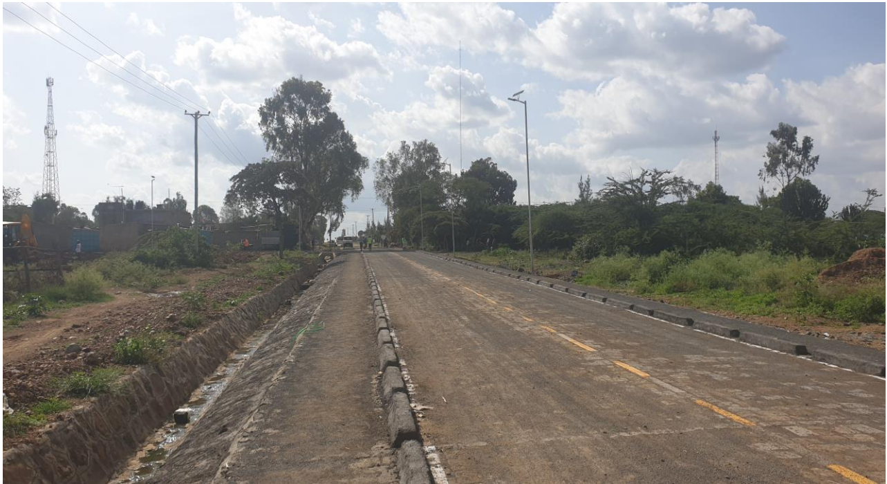
Figure 8: Well aligned and stone pitched side drain along Solomon Kiguru Road.
