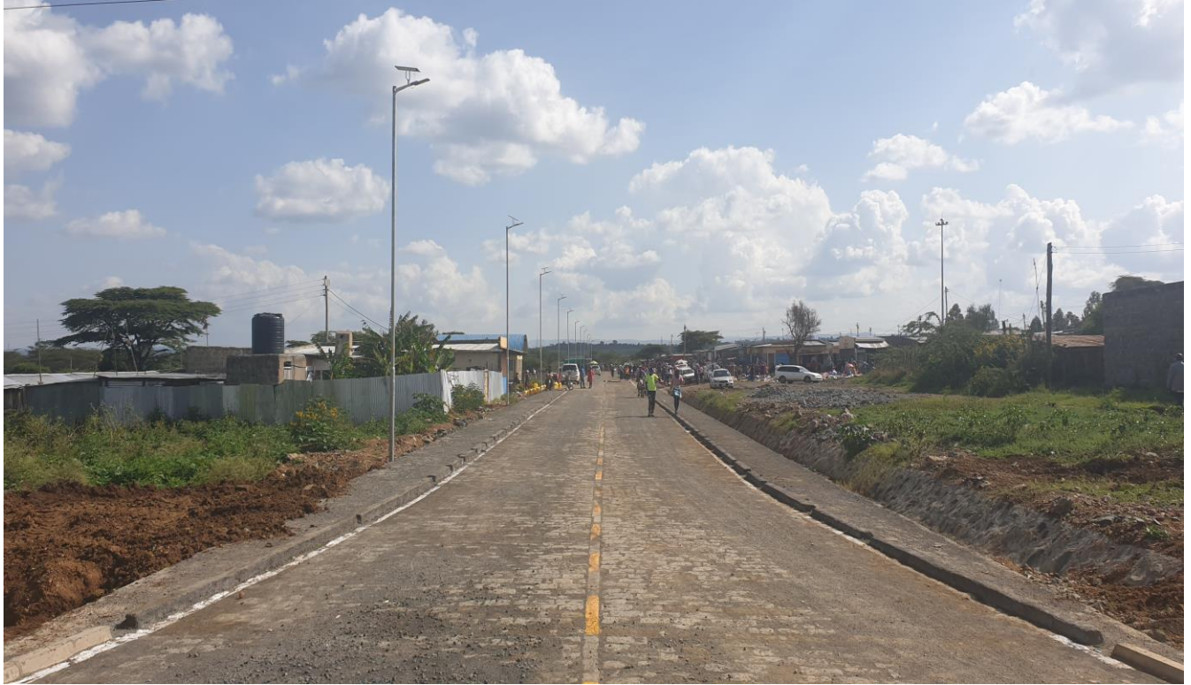
Figure 3: Completed Kihika Kimani Road.
