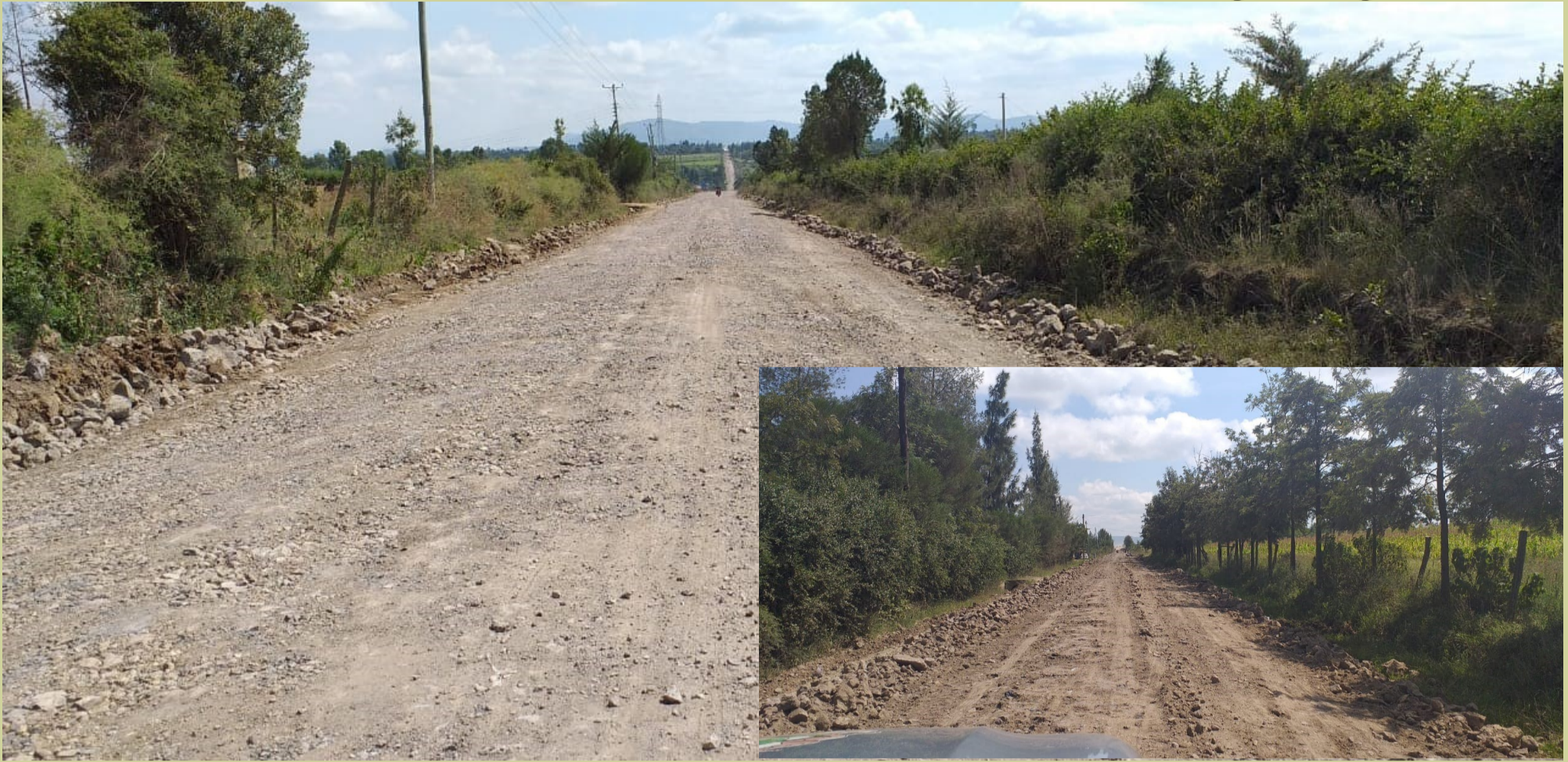
Nyarigino-Roads 2000 after compaction and (inset) before compaction
